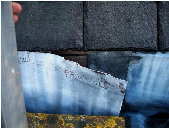
Flashing loose and falling away to south west gutter, some debris.
