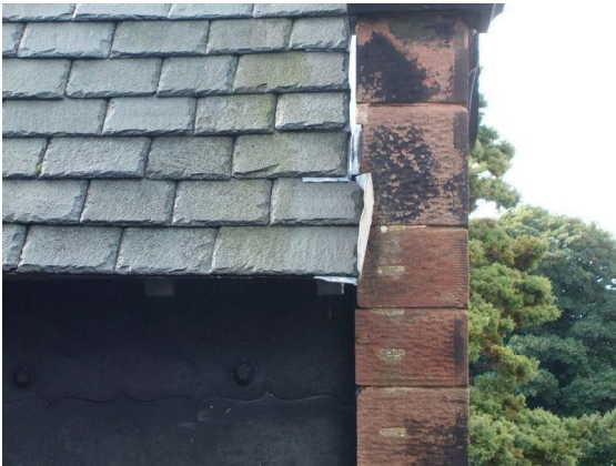
Flashing loose and falling away to south west gutter, some debris.
